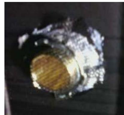
Screw lock nut over screen on the inside of overflow fitting.
